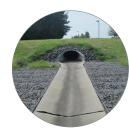
Inspect the pipe or pipes bringing water into the basin to make sure it isn't crumbling or broken. Remove any debris or dirt that may obstruct the flow of water into the basin.
